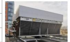
Install heat pumps
