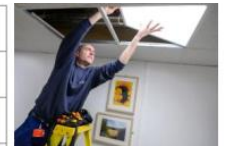
Install LED lighting
